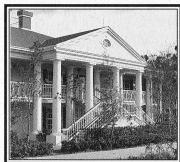
A detail of one of the many stairways at Magnolia Terrace.
